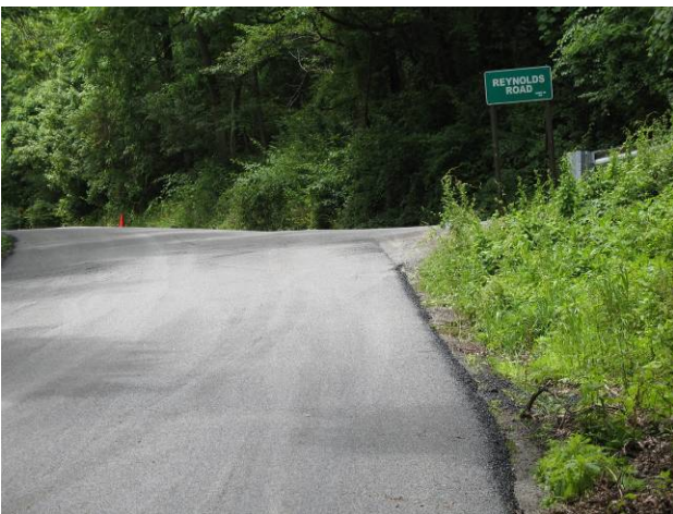
View uphill by Reynolds Road
