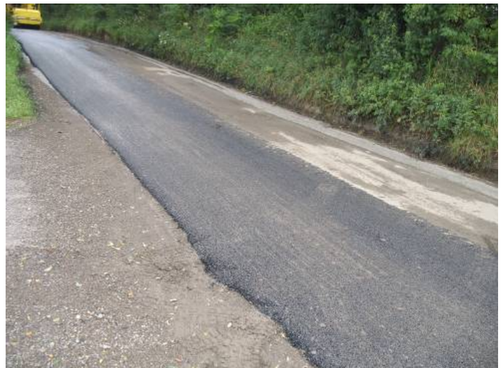
First side laid and rolled
