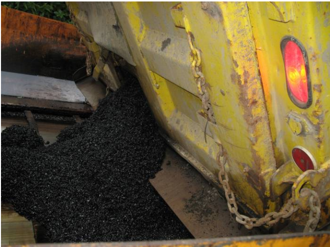
Flows through coal hole, no need to open gate
