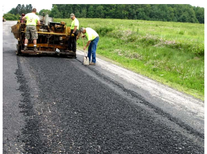
Entire crew and scratch coat
