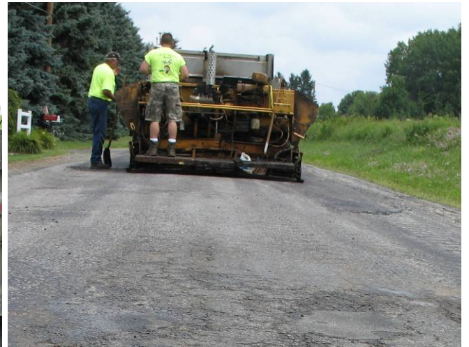
Wilson Road profile before paving
