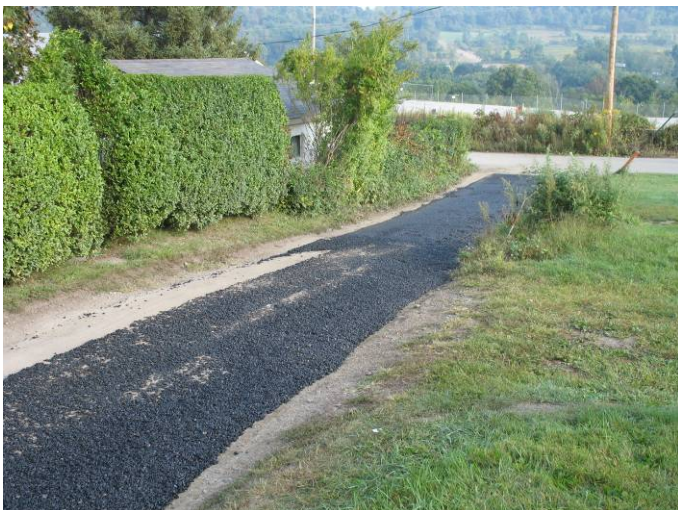
Scratch / leveling course
